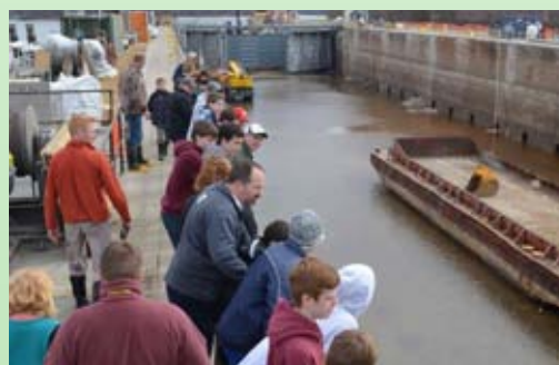
Looking down into the lock chamber. Access ports to the water supply pipe are the square openings in the opposite side. (Photo taken by Amy Bettis)
