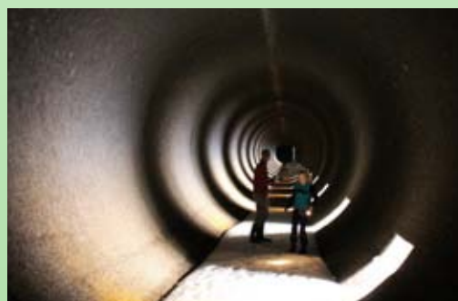
Inside the pipe. The openings we crawled through to enter the pipe are on the right. When flooded, the pipe holds 79,2799 gallons! (Photo taken by Amy Bettis)
