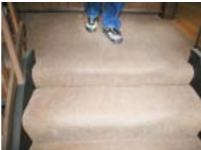
Trip hazard at top of stairs
