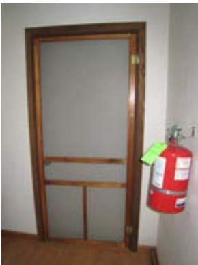
Unmarked Fire Exit to the roof & fire escape ladder
