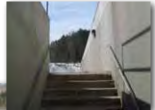
Building N, Outside exit across from Electrical Room
